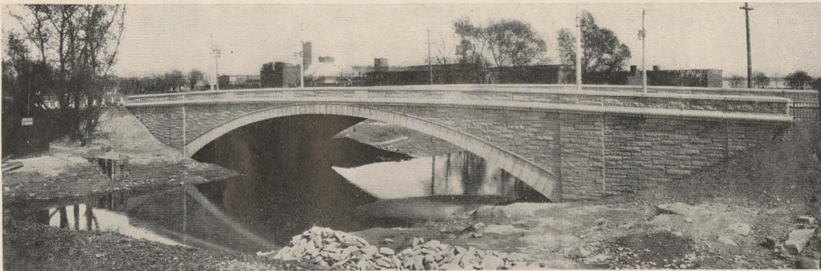
The East Fourth Street Bridge, Eddystone, Pa., erected from Mount Airy Granite CARL R. CAMP, INC., Contractor. GEORGE WRIGHT, Engineer for Delaware Co., Pa.
