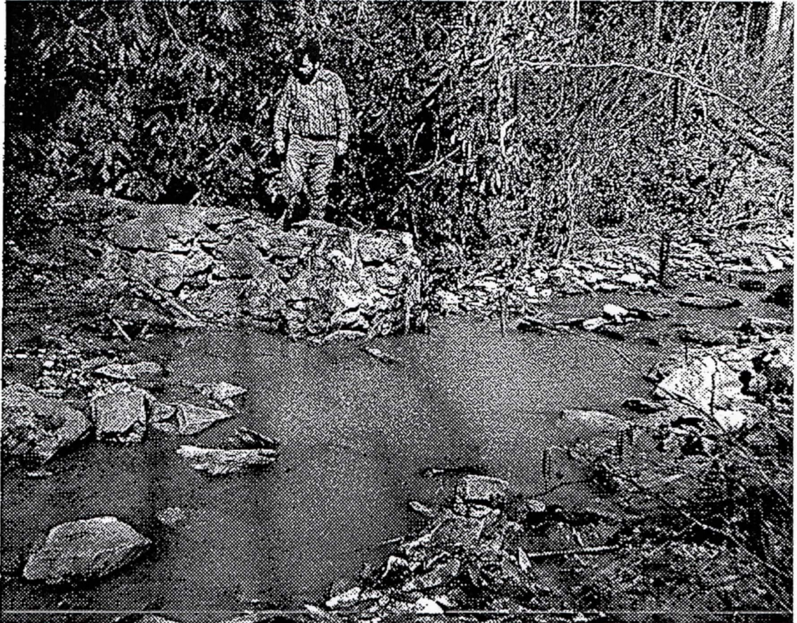
First Tumbling Rock Dam
