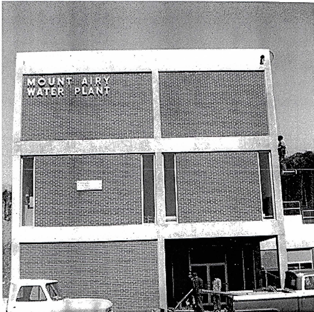
New Mount Airy Water Plant Built on Stewarts Creek
