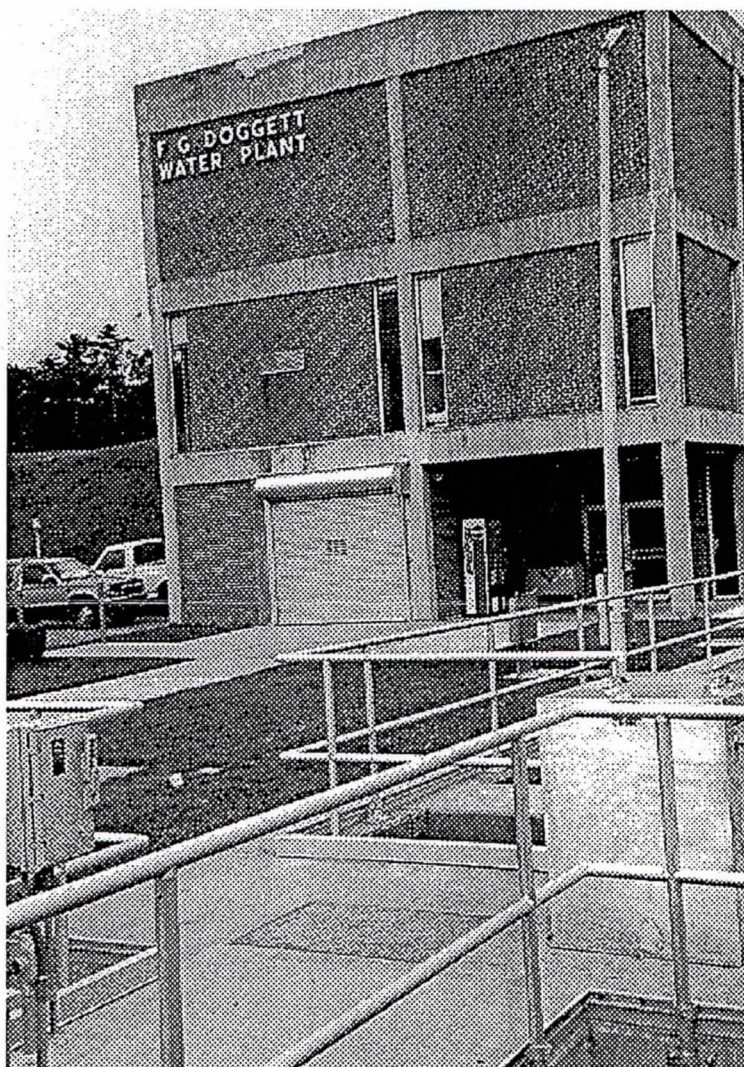
1993 F. G. Doggett Water Treatment Plant
