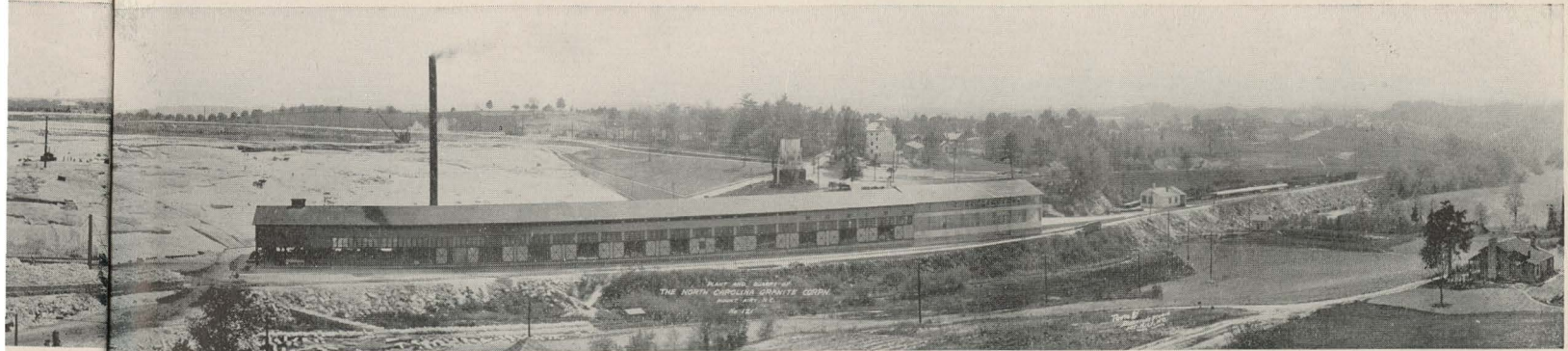
te Corp. Mount Airy, N. C. Waste has been used for roads, fills and retaining walls
