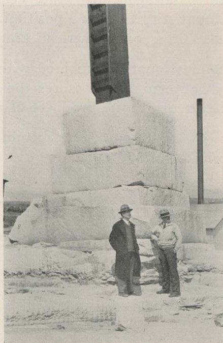
The foot of the mast is the old quarry floor. The stone blocks are segments of granite sheets loosened by "blasting" with compressed air
