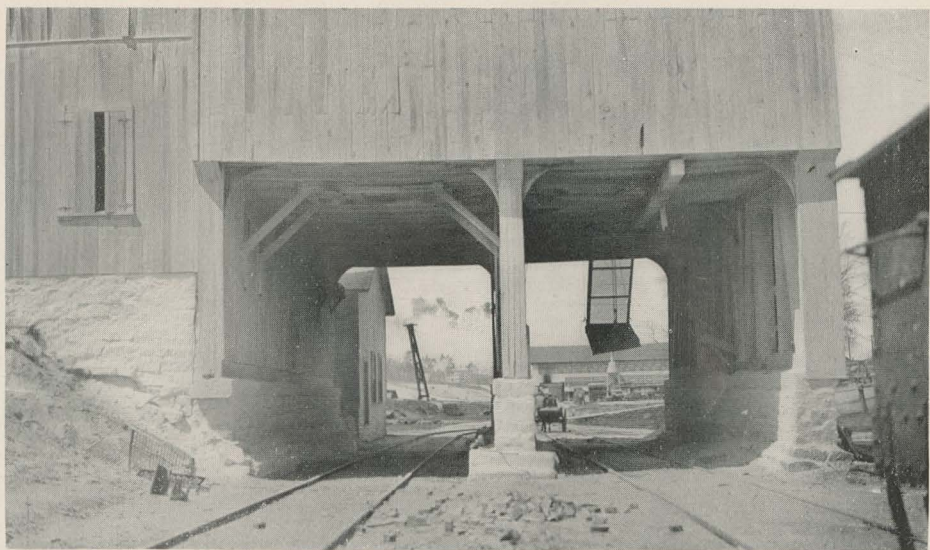
From these bins, waste granite, converted into various grades of crushed stone, is loaded for shipment
