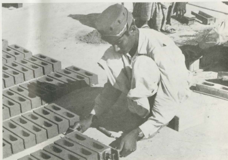
Making cement bricks for the New United Christian Hospital.
