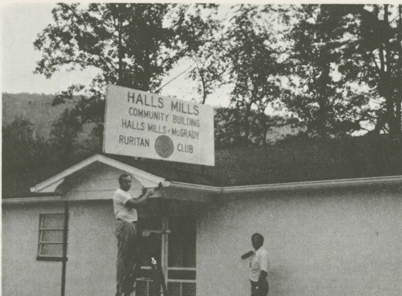
Halls Mills-McGrady Club remodeled, painted community center; also built new bathrooms. Pictured: Henry Hall, club president, on ladder; Johnny Edmiston, past president.
