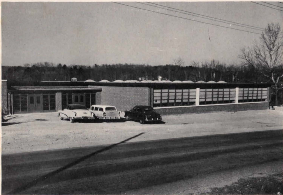
NORTH MAIN ST. EXTENSION SCHOOL
