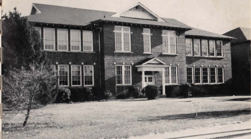
NORTH MAIN ST. SCHOOL 1955-56 Mt. Airy, North Carolina
