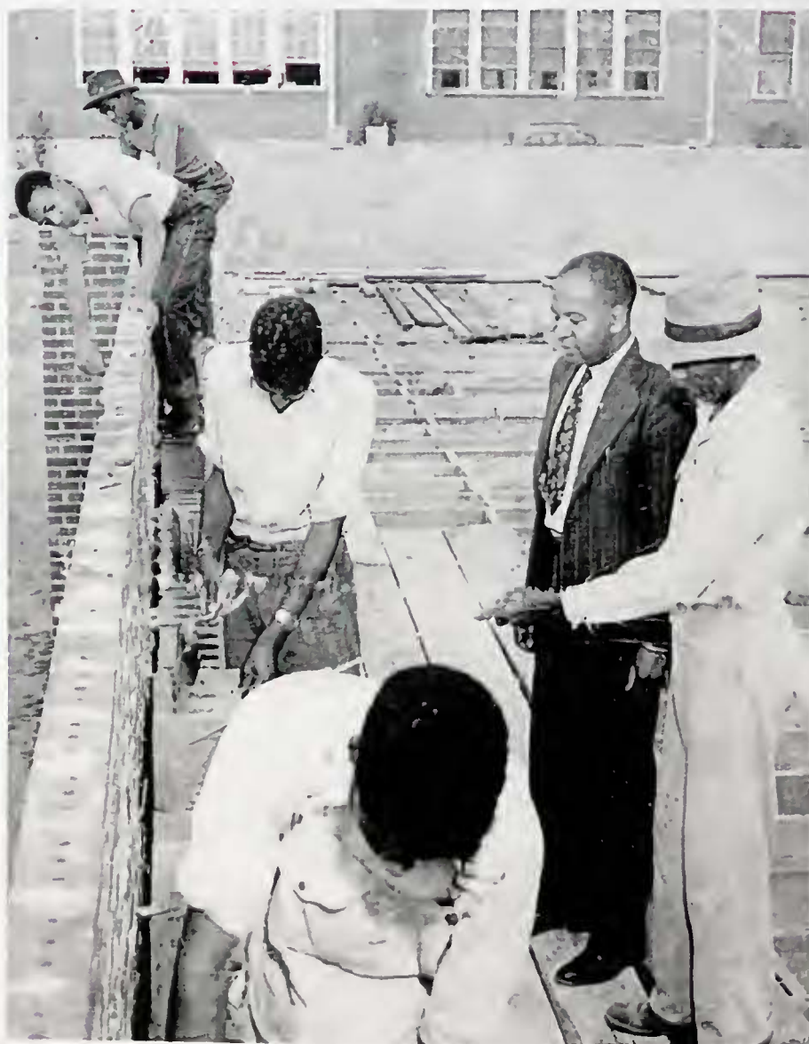
Building J.J. High School
