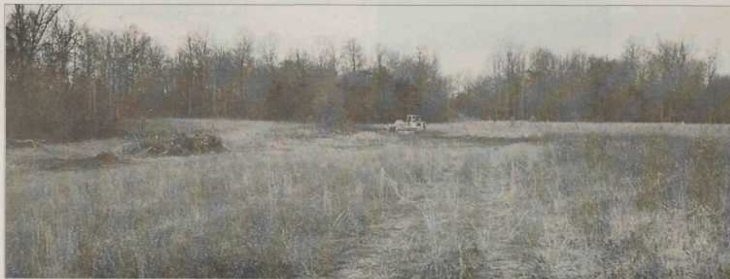
Contractors prepare to turn this pasture area into the site of a new Surry Community College classroom.
