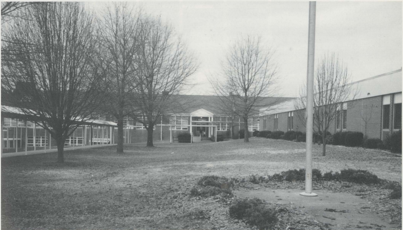
The Red Building was built in the late 1940's. It was used for grades 8-12 when Copeland was a high school. It housed the main office, Typing, Home Economics, Library, and the Cafeteria, which is still currently being used. Also in this building are grades 4 and 5, Art, Computer Lab, Guidance, Music, Hispanic, and Exceptional Children.
