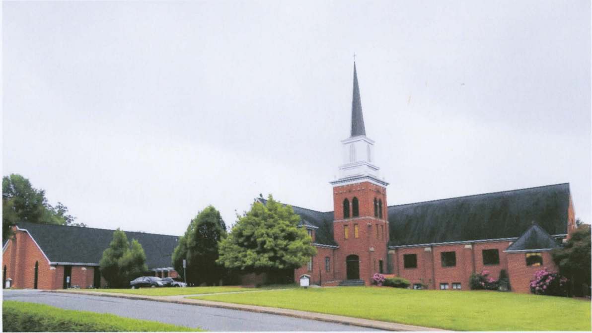
Figure 136: First United Methodist Church, 2012.
