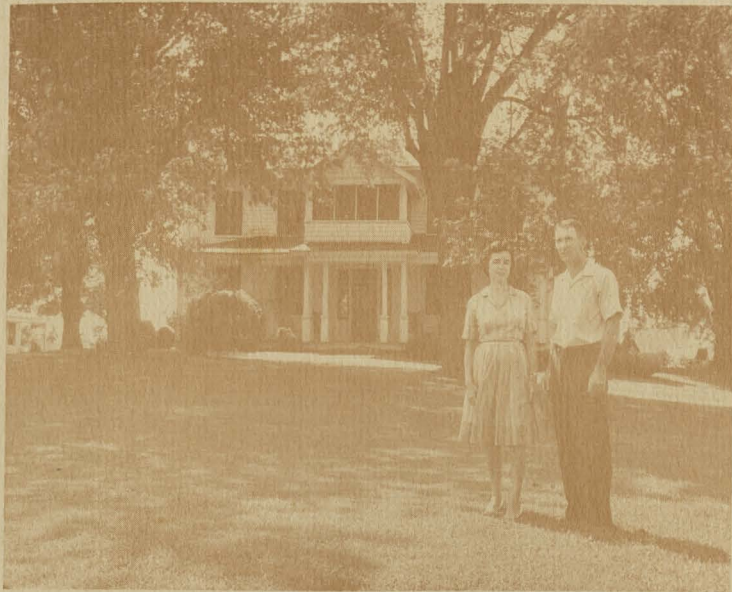
EXTERIOR VIEW OF HOME
