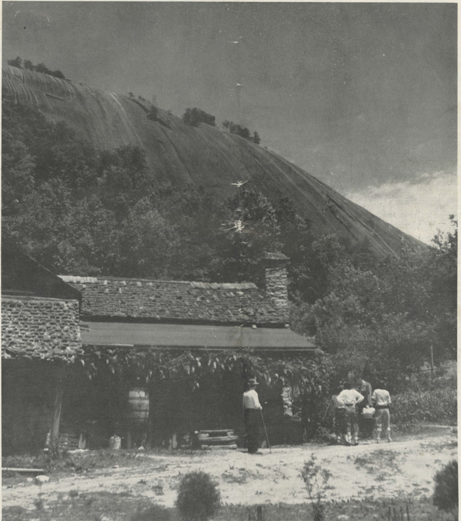
THE HUTCHISON HOME on the South side of Stone Mountain is a welcomed rest stop for hikers on the trail from Camp Butler to Stone Mountain. Stones from the mountain were used for the chimney and steps of the home. The roof shingles are hand split boards.
