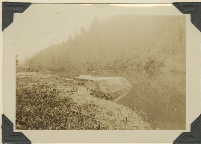
Fig. 2 Concrete Intake
