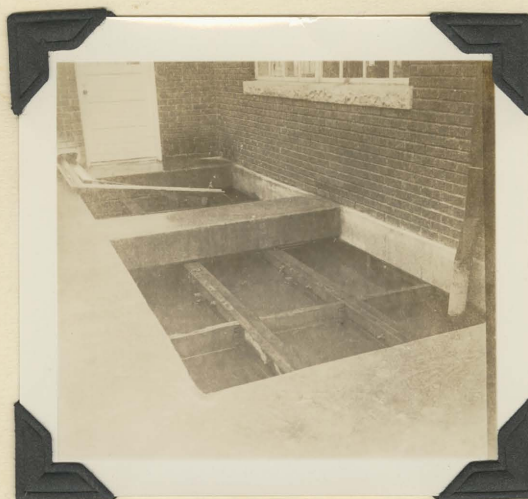
Fig. 12 Mixing Chamber
