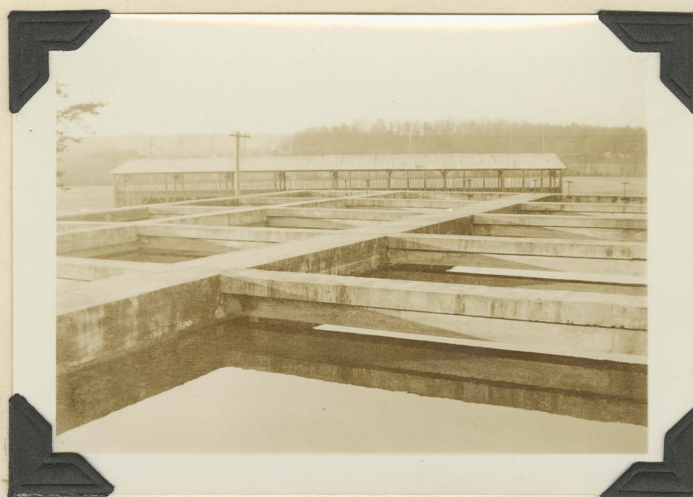
Fig. 4 Coagulation Units
