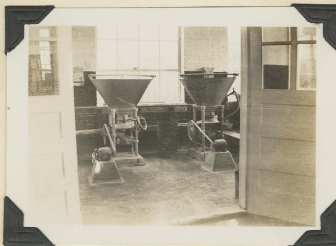
Fig. 5 Dry Feed Machines
