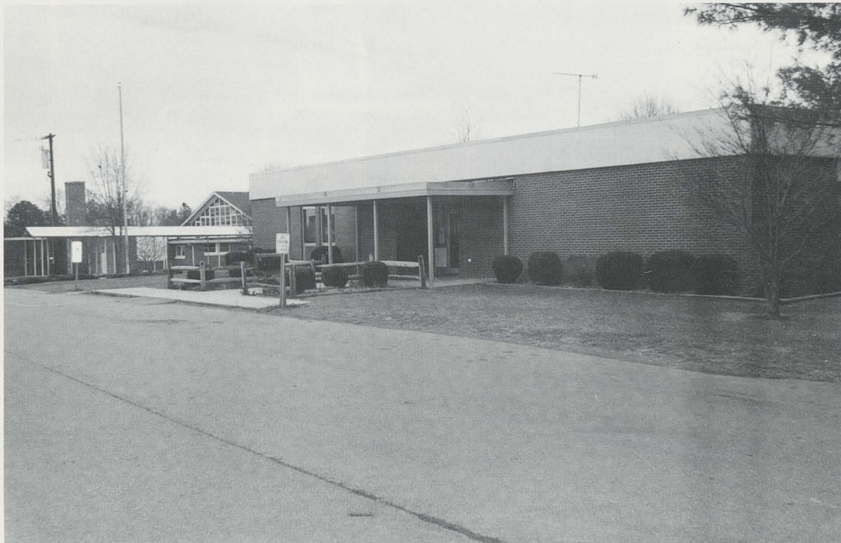
Copeland Elementary School Dobson, North Carolina
