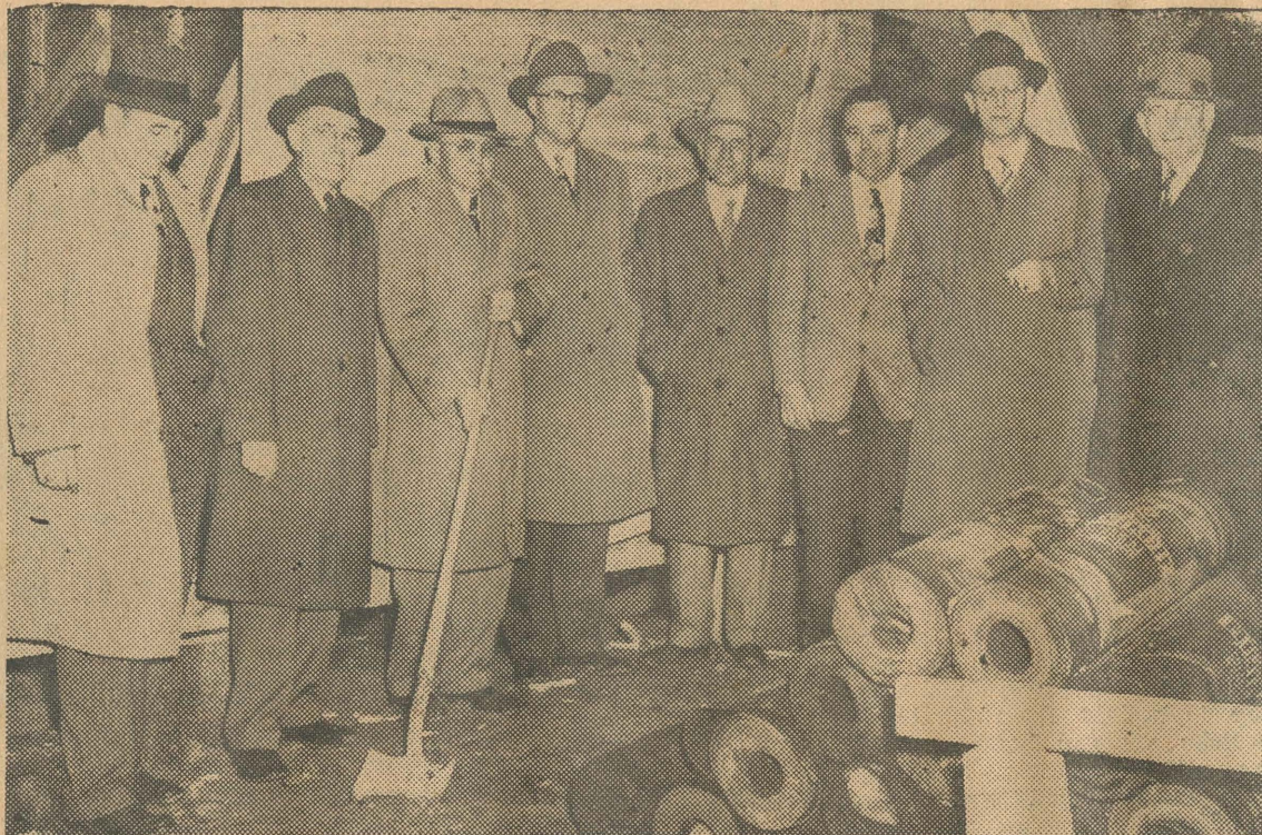
GROUND BREAKING —Officials of the Community Foundation broke ground for Mount Airy's Reeves Community Center Tuesday afternoon, January 30, 1951, in front of the tool house on the proposed building's properties. Shown for ceremony are left to right, R. D. George, Secretary-Treasurer of the Foundation; W. F. Carter, Jr., Mayor of Mount Airy; James F. Yokley, Chairman of the Foundation; Charles M. Graves, Recreational Engineer; Committeemen J. H. Crossingham, Hugh Merritt, D. C. Lewis, and J. R. Smith. (Staff Photo.)
