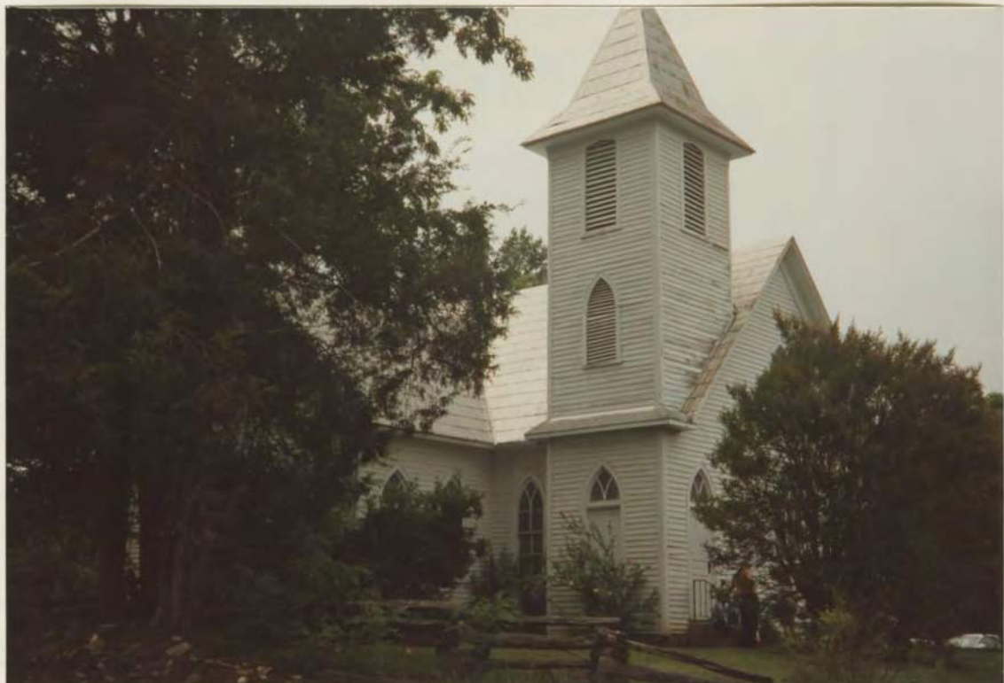
Historic Rockford Methodist Church, July 1994.
