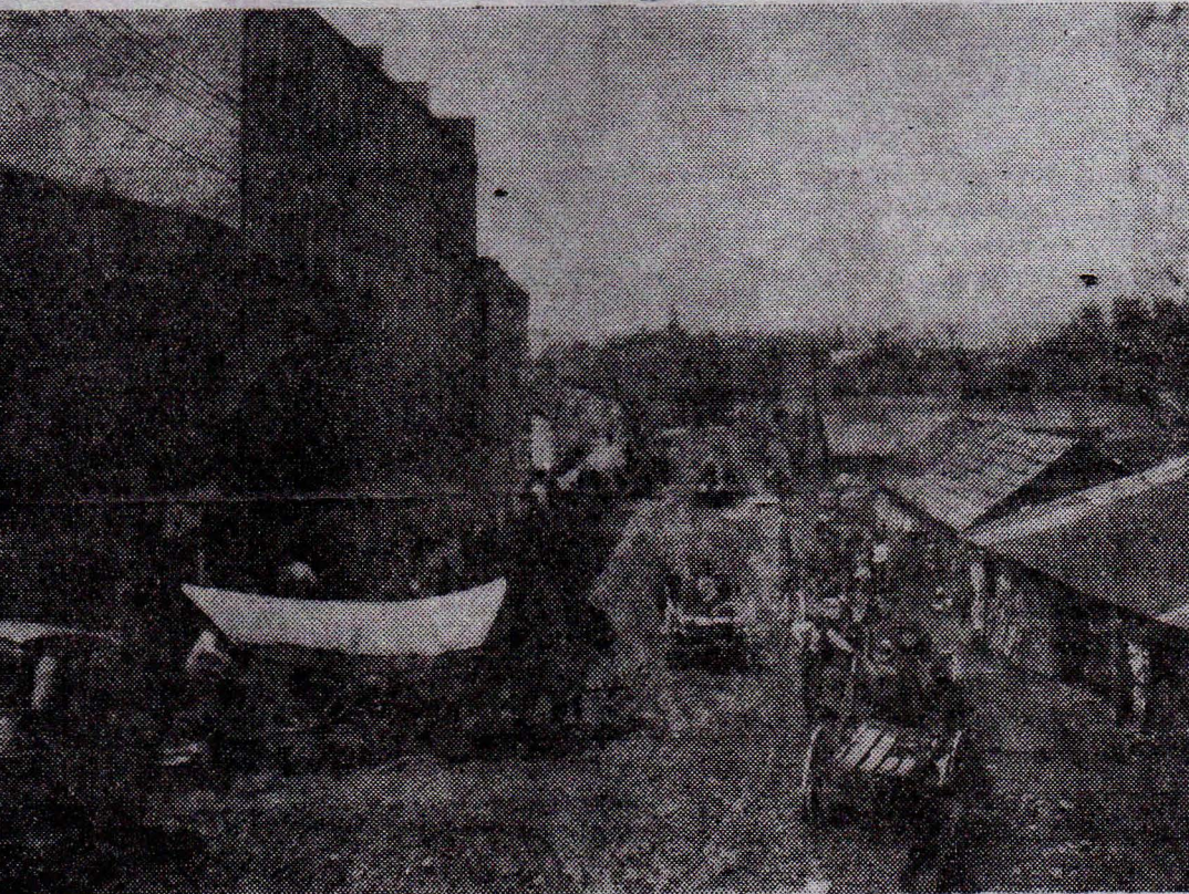
PAGE OUT OF THE PAST— Here is Virginia street, in Mount Airy, as it looked shortly after the turn of the century. The covered wagon at the left is taking on a load of fertilizer from
