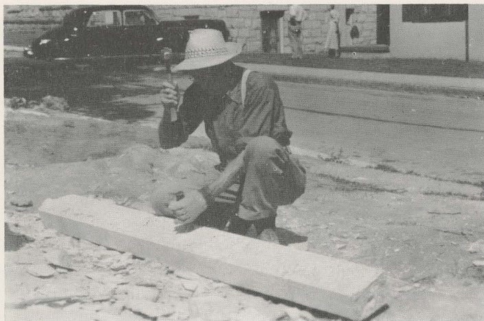
Above photograph shows how Sawed Bed Ashlar is traced before it is turned over and knapped with a hammer into desired lengths.
