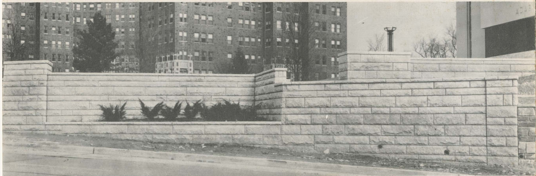
Approach walls at Adas Israel Congregation, Washington, D. C. Built of Mount Airy Sawed Bed Ashlar by Louis Perna Stone Company.
