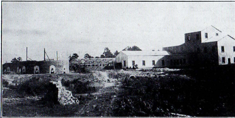
NEW $200,000 BRICK PLANT OF THE SHALE BRICK COMPANY, SANFORD, N. C.
