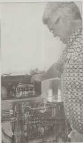
Mike Tolson checks the equipment that will be the circuitry being installed in the Reeves Building at Barry Community College.
