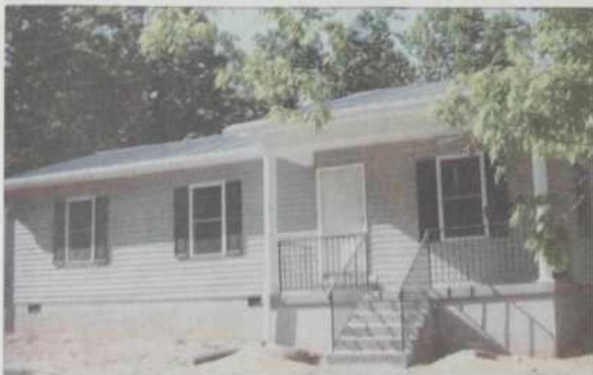
The Yadkin Valley Habitat for Humanity home in Thurmond was built by students in the Construction Trades Program at SCC.
