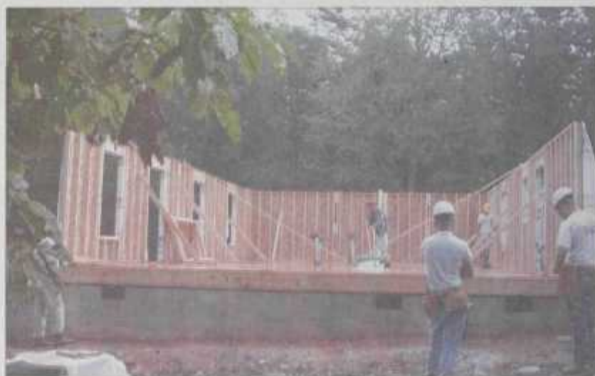
Work on the house for the James Martin family began in 2004.
