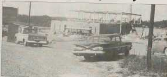
Construction continues on the first building at Perry Community College in the 1940s photo. The college received a 14th building this year.
