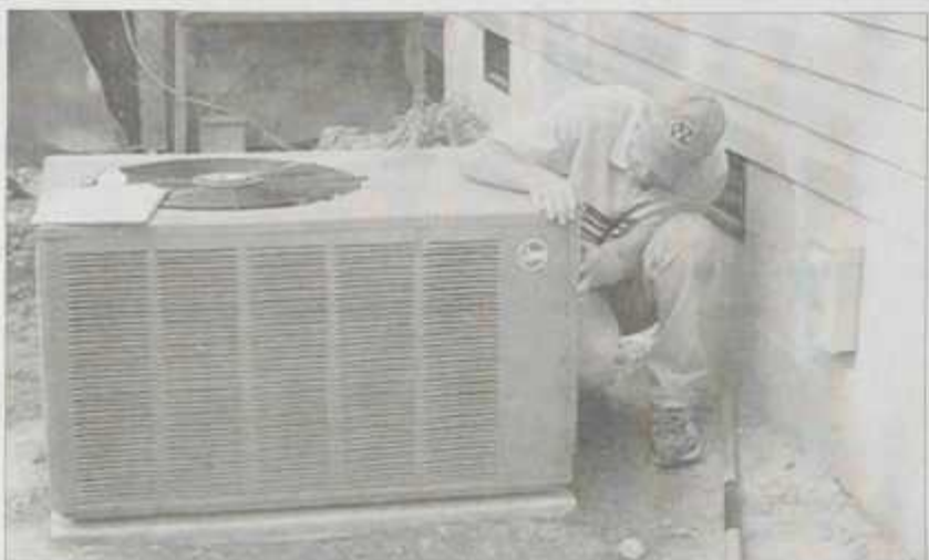
Brian Chilton works on the home's AC unit.
