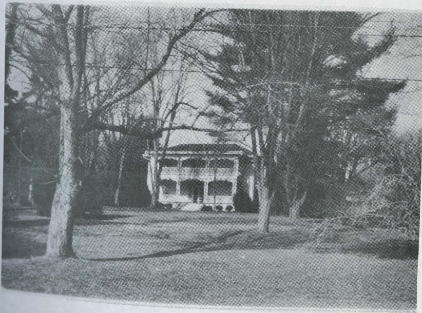
This handsome structure in the heart of Elkin was built in the 1850's, the home of Richard Ransom Gwyn. General Stoneman, of Civil War fame, is said to have stopped here.
