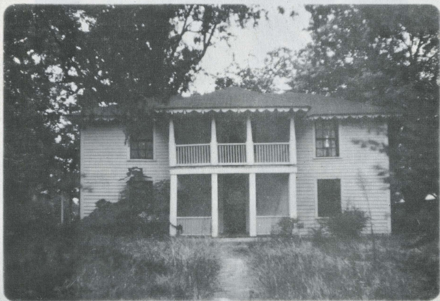
Colonel Waugh house, presently known as the Llewelyn house in Dobson. It was supposedly built just after the Civil War.
