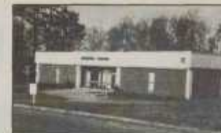
Electronics building - Electronics building opened in 1988 (to be renovated in 1998-99).
