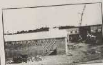
Shop building and T building under construction - 1966.
