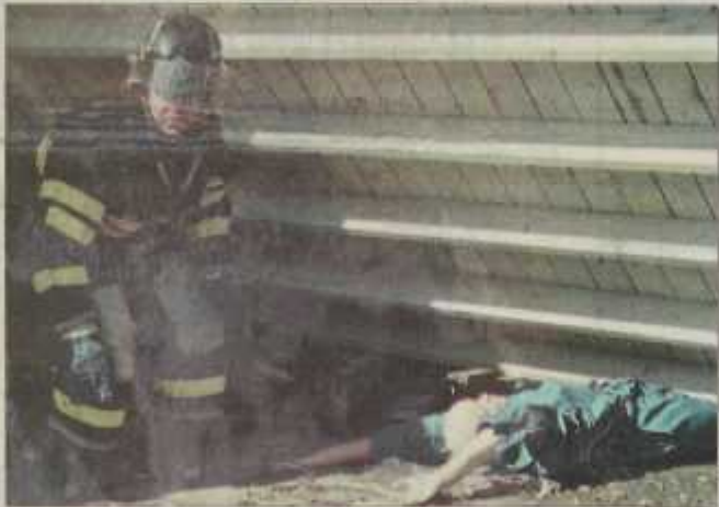
A member of the Dobson Rescue Squad prepares to help remove a rescue dummy from under the collapsed roof of the Elmore's building.
