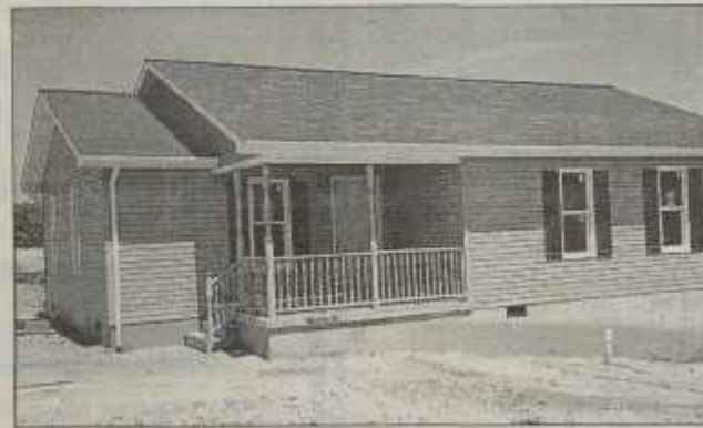
THE COMPLETED PROJECT —This is the home of Craig and Lisa Smith at 105 Robin Street, Boonville. It was built by students from Surry Community College in partnership with the Upper Yadkin Valley Habitat for Humanity. (Lynn Templeton-Photo)
