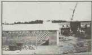
Shop building and T building under construction - 1966.
