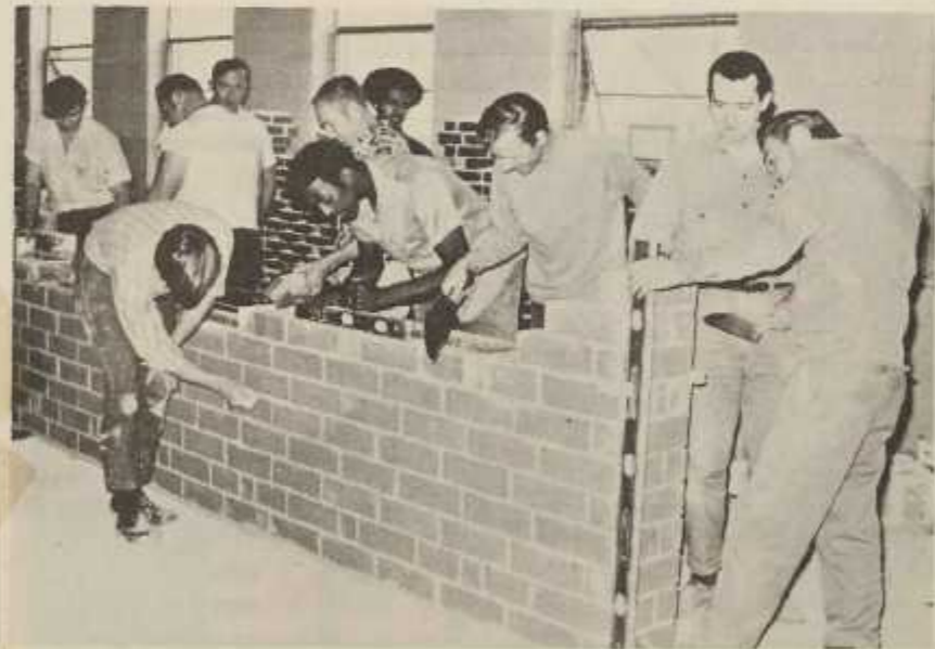
A FULL-TIME BRICKLAYING COURSE is conducted at Surry Community College with the aid of a Federal grant. Students are shown putting the finishing touch on one of their projects.
