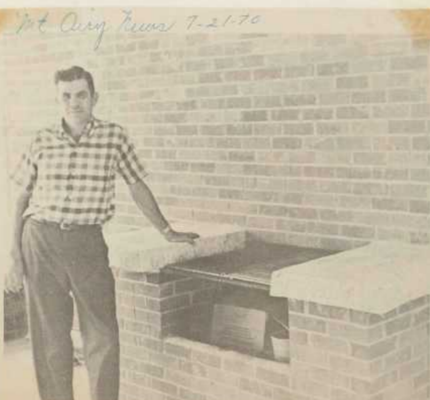
SIXTEEN ADULTS HAVE COMPLETED a masonry course at Surry Community College. They include: Phillip Anderson, William Brown, Danny Rowman, Dillard Bullin, Howard Carpenter, Samuel Collins, Carl Dalton, Donnie Dalton, Caley Easter, Roger Rapten, Robert Harris, Robert Kincaid, Danny Leonard, William Puckett, Donald Slate and James Slate. Showabove, Greater Haymow, instructor, is pictured inspecting the live project which the class completed prior to graduation from the course.
