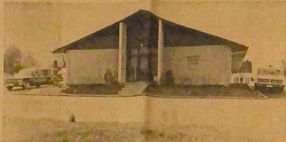
The new and modern Moody Funeral Home and Chapel, located on Kapp Street in Dobson, will be formally dedicated in service scheduled Sunday. Open house will be held from 10 a.m. until 10 p.m., and dedication services are scheduled at 4 o'clock in the afternoon.
