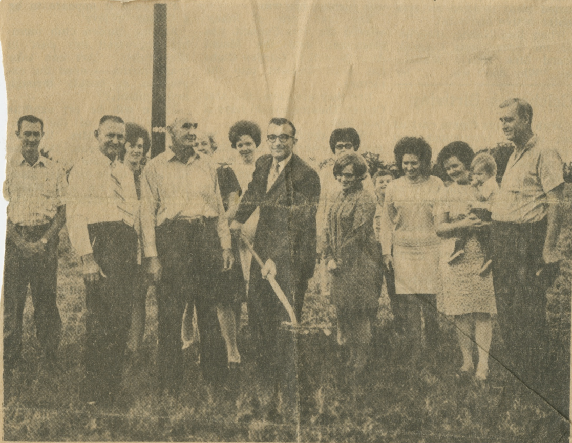
... Joe Brown and Boyd Brown, deacons, join Pastor Adams for the groundbreaking...
