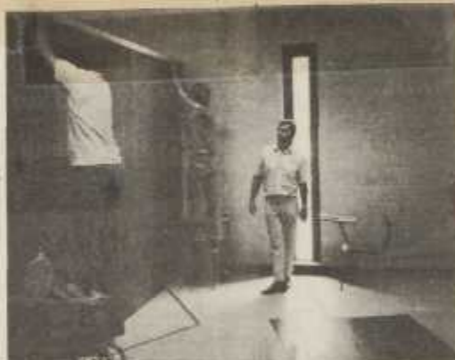
INSTRUCTOR BILL HATT and students at Surry Community College study basic building skills.
