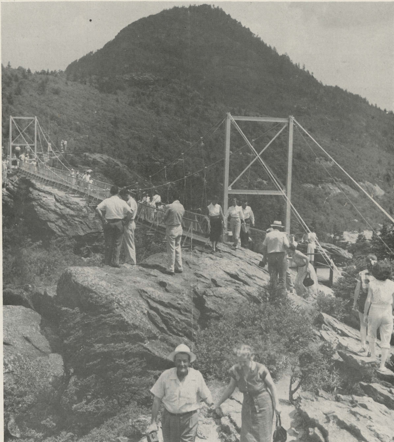
THE ERECTION OF THIS SUSPENSION BRIDGE between the two higher peaks on Grandfather Mountain near Blowing Rock has induced many thousands of tourists to visit this scenic wonder each season. The view from these peaks is a scene never to be forgotten, and in October the autumn foliage on this and surrounding mountains will be a vast and colorful panorama. (Photo by Walt Burgiss)
