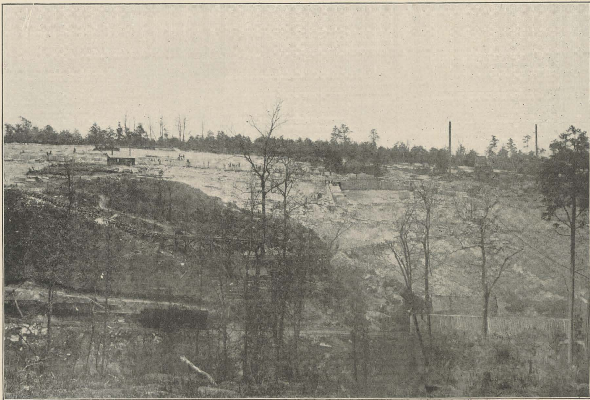
Mount Airy Quarries—General View of a Worked Portion.
