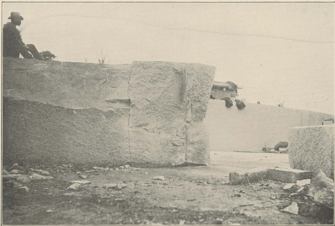
Mount Airy Quarries—Main Quarry, the Lifting Process.
