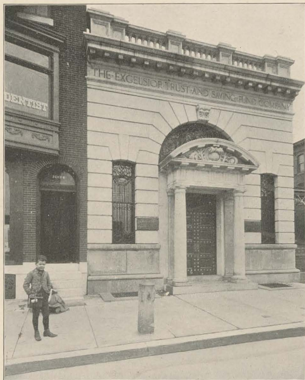
Mount Airy Granite in Use—A Bank Building, Lehigh Avenue, Philadelphia.
