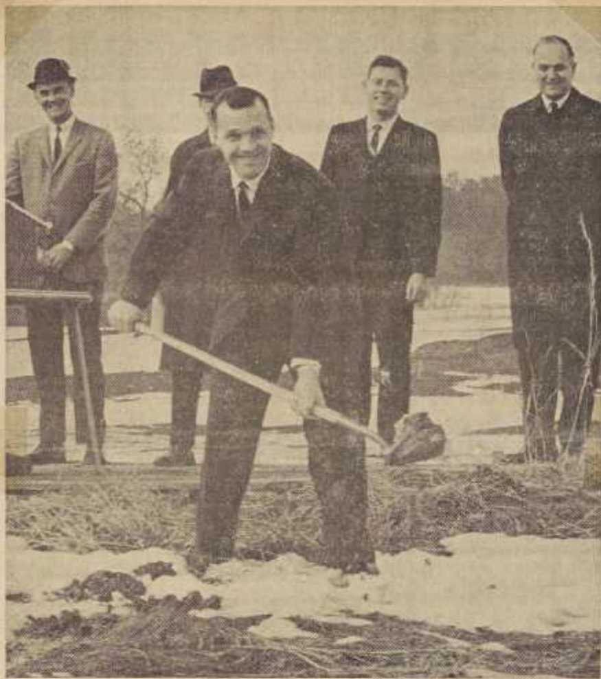
THE BEGINNING —Robert Merritt turns the first earth in ground-breaking ceremonies at the site of Surry Community College. Merritt, vice chairman of the college's board of trustees, performed the act instead of Chairman Robert Burrus, who was ill and unable to attend. In the background, from left, are Jack Folger, trustee; the Rev. Donald Davis, who brought the invocation; and I. John Krepick, college president.
