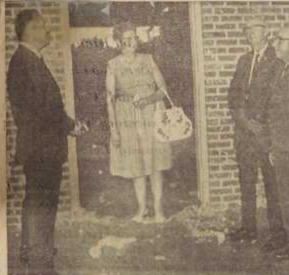
INSPECTING COLLEGE—L. John Krepick (left), president of Surry Community College, conducts members of the Board of Trustees on a tour of the college building site. The trustees are, from left, Mrs. Roxie Roth, W. I. Munday, Robert S. Burrus, H. O. Woltz Jr. and Charles L. Folger.
