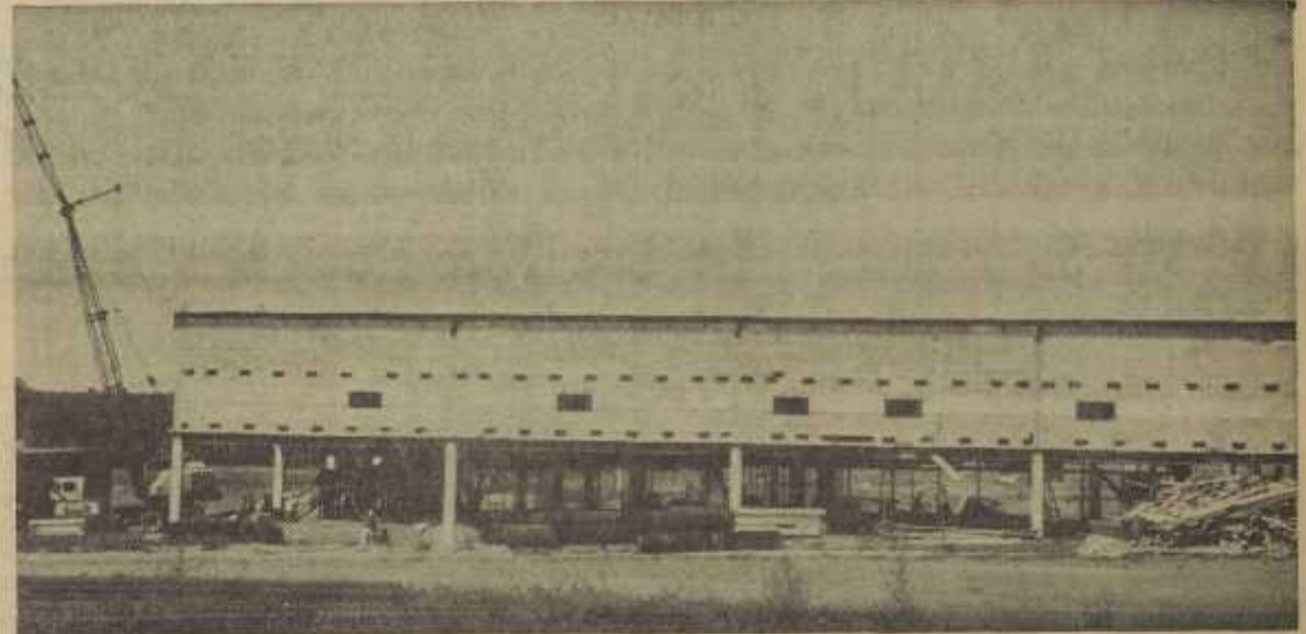
SCIENCE-TECHNICAL BUILDING STANDS AS IF ON STILTS
