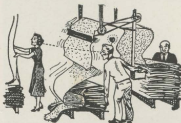
WINDING METALLIC CLOTHING — K. A. Walters, Shop, shown at left, and Eugene Powers, Wool Room No. 2, center, are receiving instruction from Ernest Eura of Ashworth Brothers, Charlotte, on winding metallic clothing on grooved cylinders. Cylinders have previously been sent out from this operations but it is now being done in the Shop.
