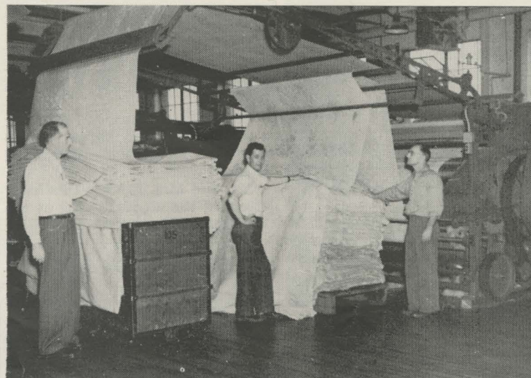
OVERSEER PAGE BRANNON, left, ROBEY PINNIX and LEE PINNIX are watching the operation of a tandem napping machine as it raises the fibers on a foxy-looking blanket in the Napping Department. (Staff Photo)
