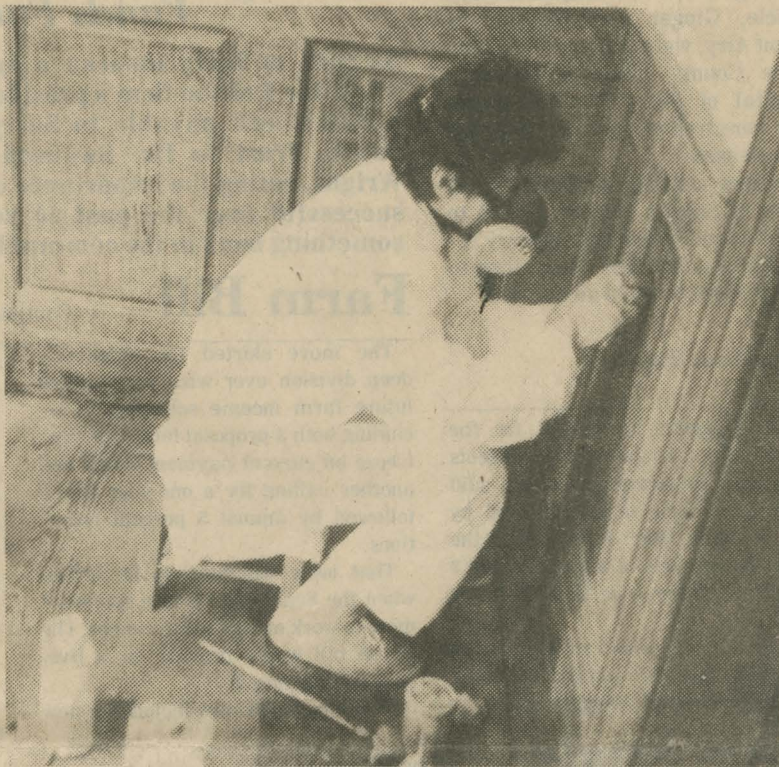
Nancy Hyne works to restore kitchen woodwork.
