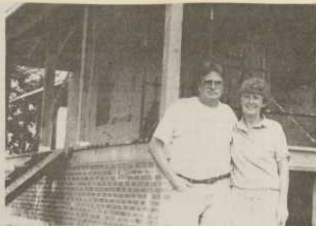
Dorothy and Skip Price stand in front of their home which is being built by the Surry Community College construction class. They hope to move in by November. (Staff photo — Palmer)
