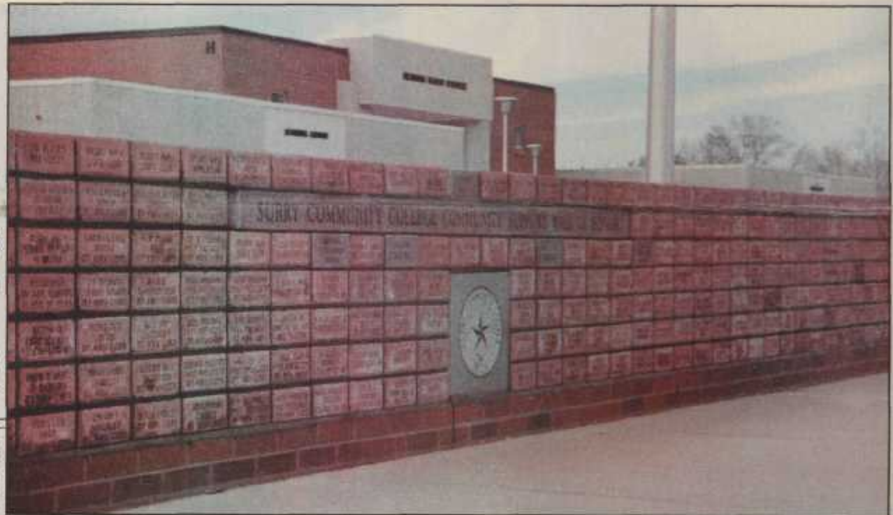
Amber Wood/The Mount Airy News THANKS TO ALL: The Wall Of Honor at Surry Community College honors supporters of the college with engraved blocks bearing their names. SCC has been engaged in several construction projects recently. Read more about them in stories on page 3 and 4.
