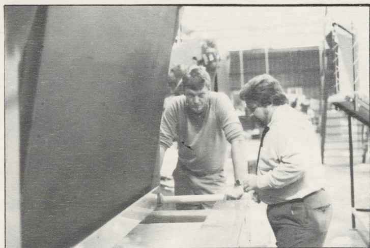
John Quwang was one of the Danish erectors to help the operation start. John and Dennis Burton, shift supervisor, watch as the garnetted fiber enters the weigh pan.
