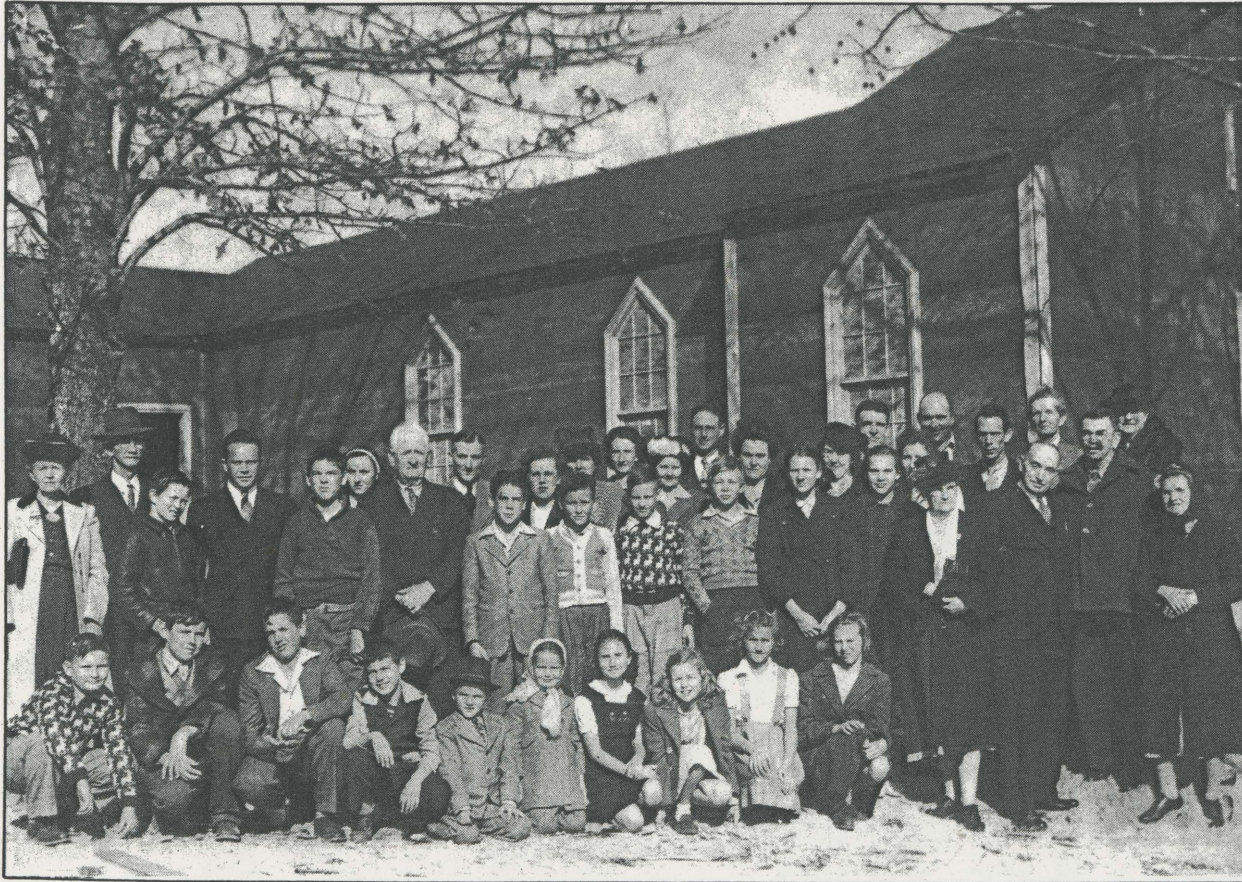
Members of the Mount Airy Church of Christ, known as the Highland Park Church of Christ, pose in front of the old church building on U.S. 601 in a photo taken in 1946.
