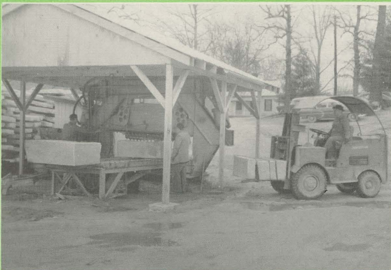
Curb Splitting Machine in Operation
