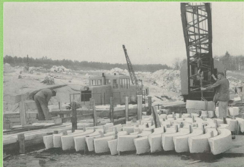
Loading Radius Curb on Flat Car
