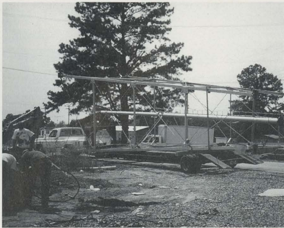
New replaces old. This water tower served us well.
