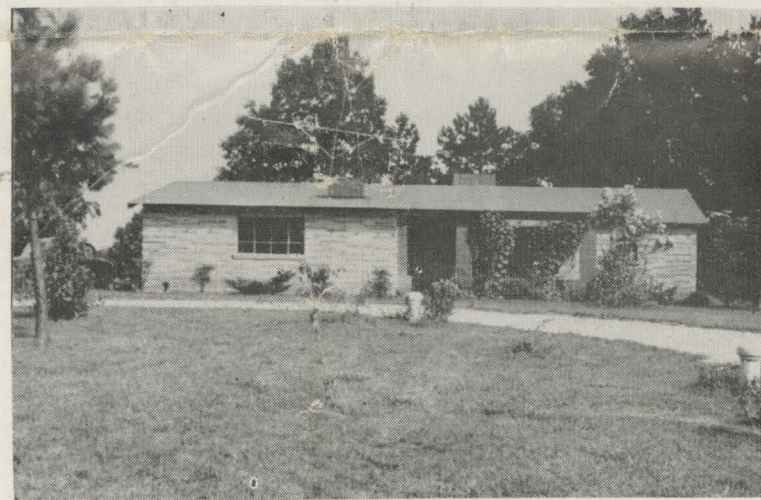
THIS ATTRACTIVE RANCH TYPE RESIDENCE is the home of Mr. and Mrs. Paul Kennedy, and is located on Oakland Drive just a short distance from Highway 21. Paul is Foreman of Burling No. 2. (Staff Photo)
