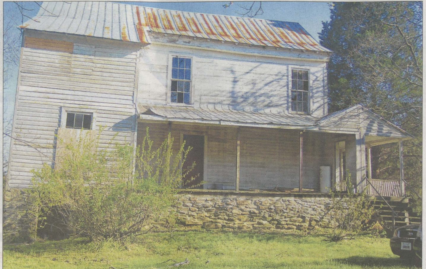
The former William P. Dobson store, built around 1813 in Rockford, was one of the dominant buildings in the town, serving as a general store along with a meeting house. Here is a photo from the structure before restoration work began about a decade ago.
