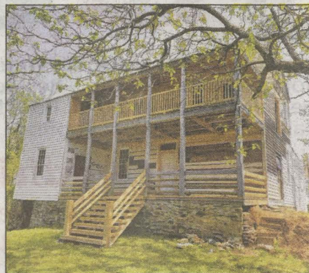
This photo shows the building in the midst of outdoor renovations, with new railings on the front porch and deck. (Photo courtesy Hannah Holyfield)
