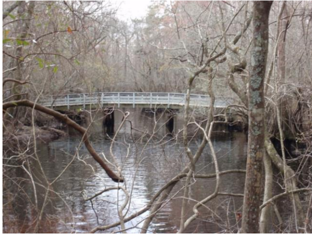
Bridge over Moore's Creek
