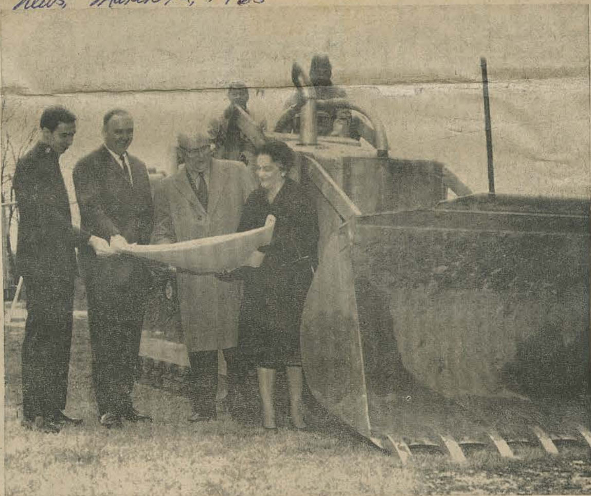
GROUNDBREAKING TAKES PLACE the easy way on the site of the new Salvation Army Citadel on South St. Dennis Moody sits in the driver's seat while Jack Greenwood gives operating instructions. Viewing the building plans are (l-r) Lt. Cecil Brogden, Gary Pruett, W. E. Merritt and Mrs. Joe Jackson. —NEWS Photo
